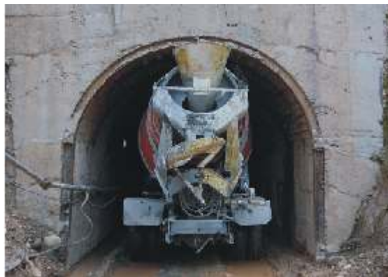
Nimo in Tunnel application
